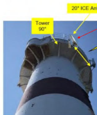
Photo montage sector B
