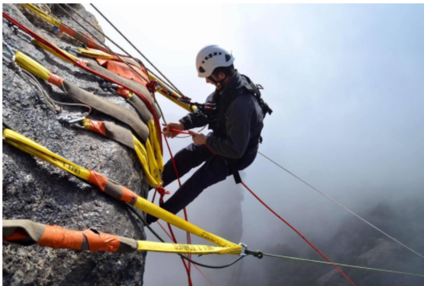
Example of 6 anchors on upper part in our Rope Jump installation
